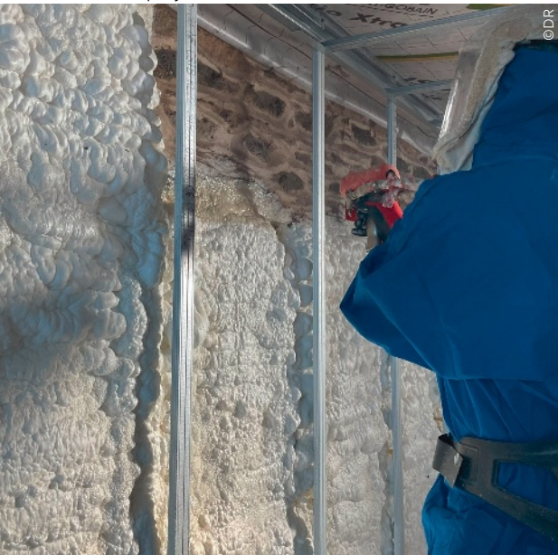
Chantier projection isolation
